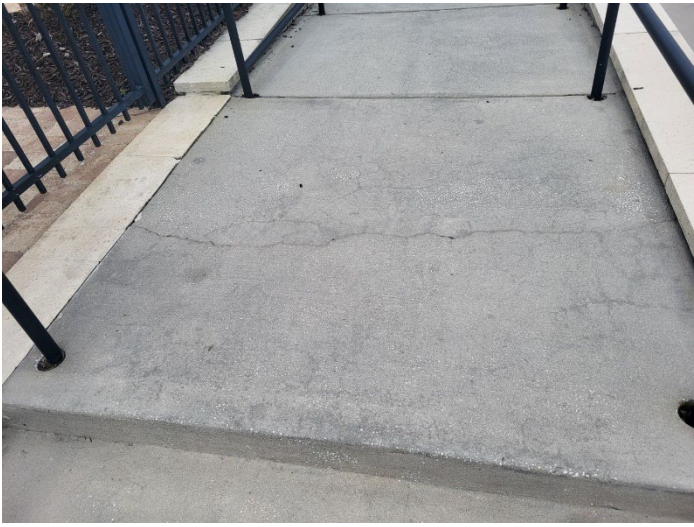
Location 1: Photo showing surface cracking of concrete at the entrance/exit gate to pool.
